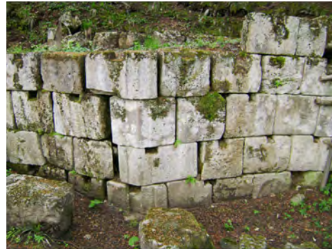
Fig. 5. Stone walls built in the opus quadratum technique. 1. Cape Sounion/Greece; 2. Dacian fortress at Costești-Cetățuie; 3. Grădiștea de Munte (photos: 1. M. Egri; 2-3. A. Rustoiu).
