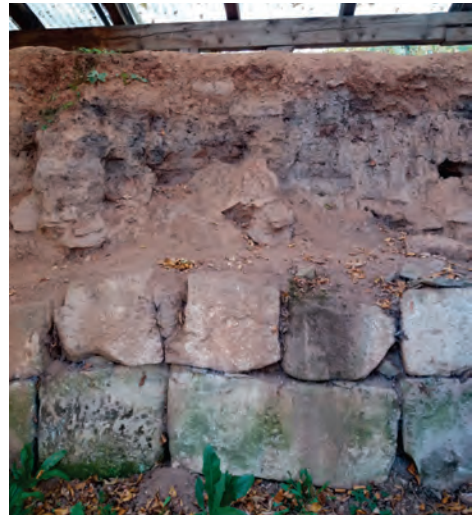
Fig. 10. Tower dwelling with the upper floor built of mudbricks. 1-2 – Costești: tower no. 1; 3-4 – Tilișca: tower no. 1; 5 – Tilișca: entrance of the tower with traces of the timber door mounting system on the threshold (photos A. Rustoiu)
