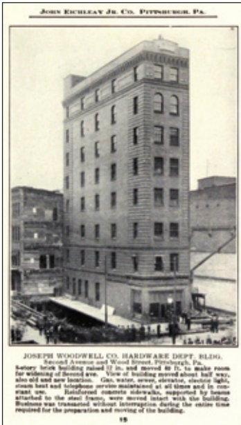
Figure 2. The Joseph Woodwell building in Pittsburgh being moved in 1921. Source (accessed in November 2018): https://www.swanngalleries.com/ms/Sale2426/lot316
