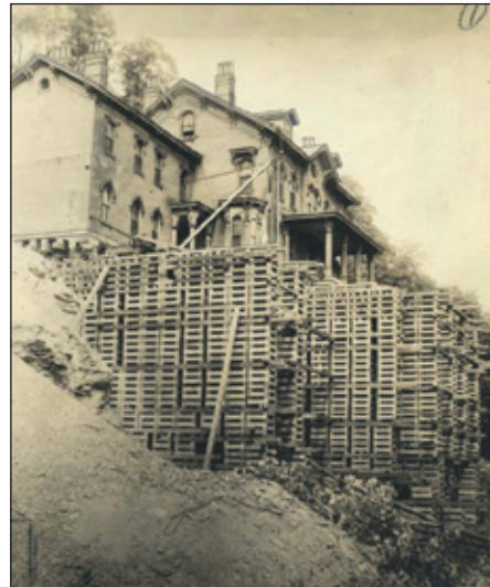
Figure 5. The house of Captain Brown being lifted in 1903. Source (accessed in November 2018): https://historicpittsburgh.org/islandora/object/pitt:20160223-hpichswp-0006/from_search/-46
