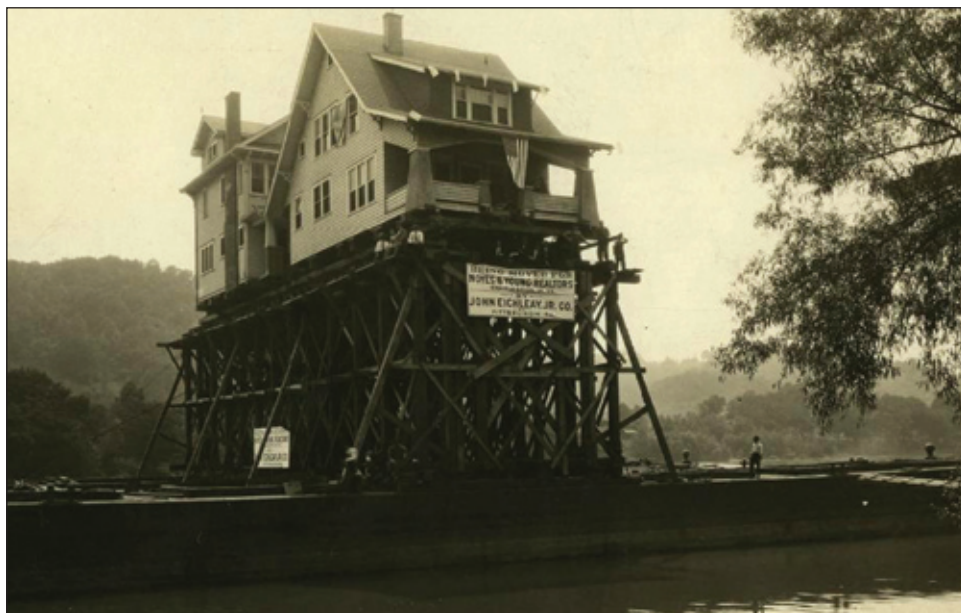
Figure 6. The Eichleay Company moving houses on a river using barges in 1921.
