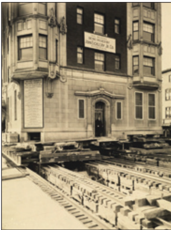
Figure 4. The Fort Frederick residential building in Albany, New York being moved in 1926.
