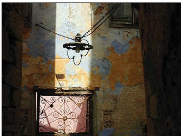
Fig. 8. A ruined wall. Chania (Greece)
